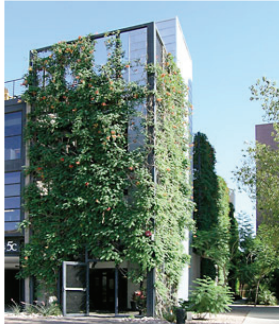
Above: Large green walls shade a south and west exposure. Source: greenscreen®
