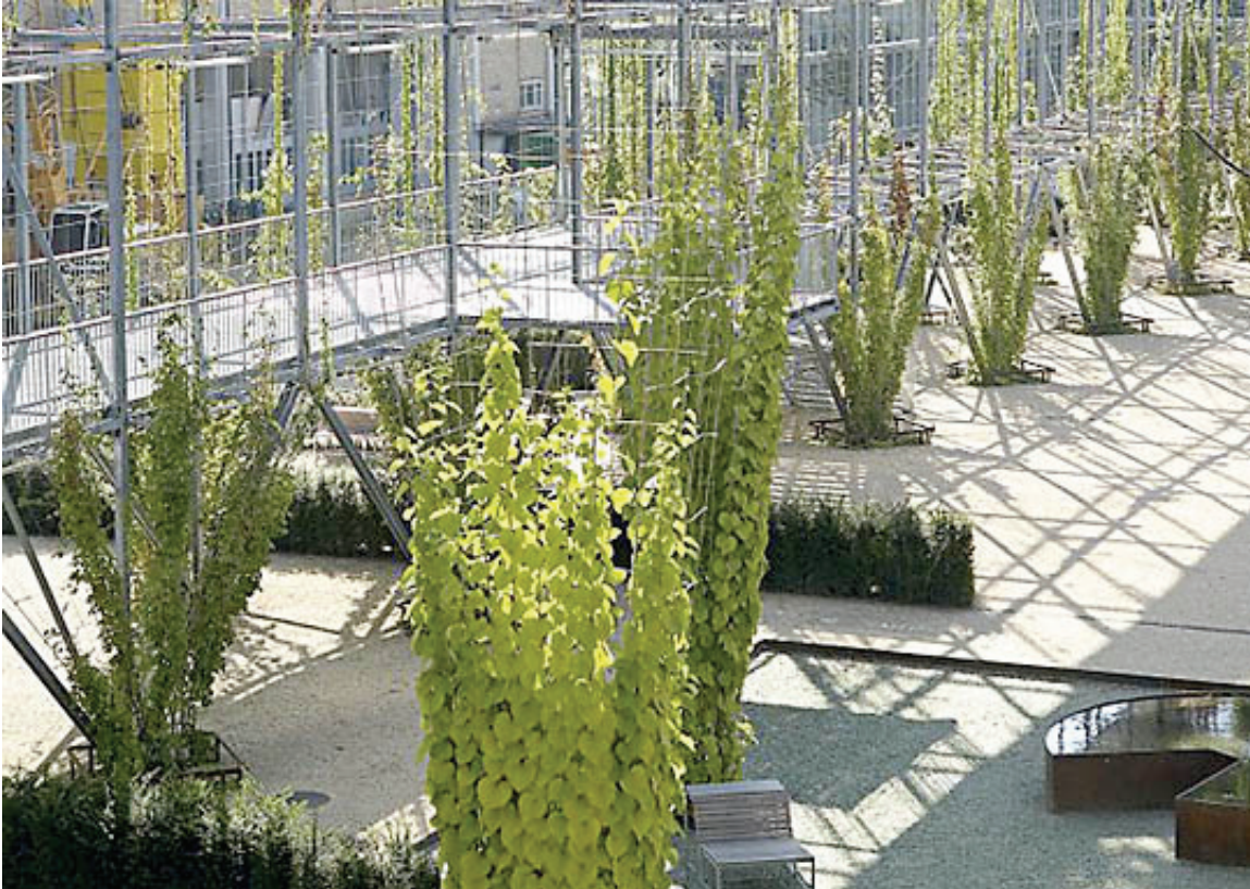
Above: Cable system example using vertical cables to create shapes. Note cables protruding up from plants and additional horizontal cable supports. Source: Jakob
