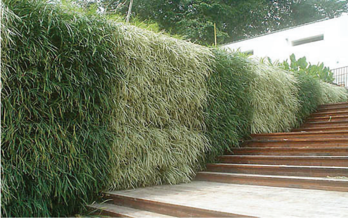
Above: A mature Modular Living Wall. Source: Elevated Landscape Technologies Below: A diverse plant selection being pre-grown for a modular living wall installation. Source: Green Living Technologies
