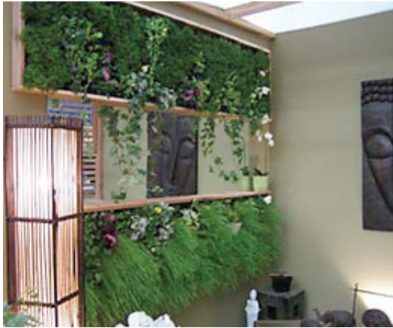
Left: A living wall constructed from modular pre-grown panels installed in an interior patio. Source: Elevated Landscape Technologies
