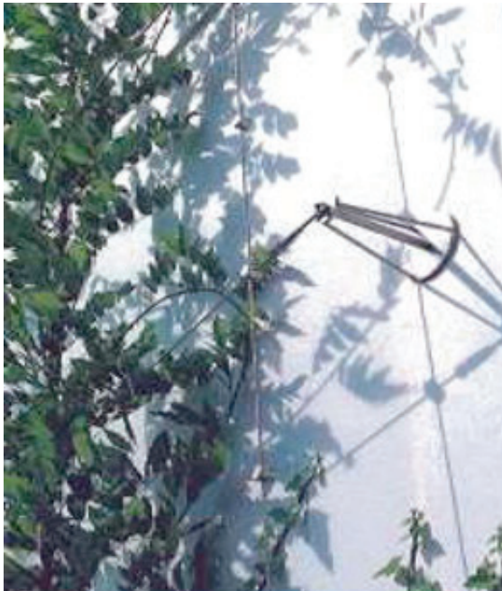
Above left: A cable system green wall may need adjustment as the plant material matures. Source: Jakob
