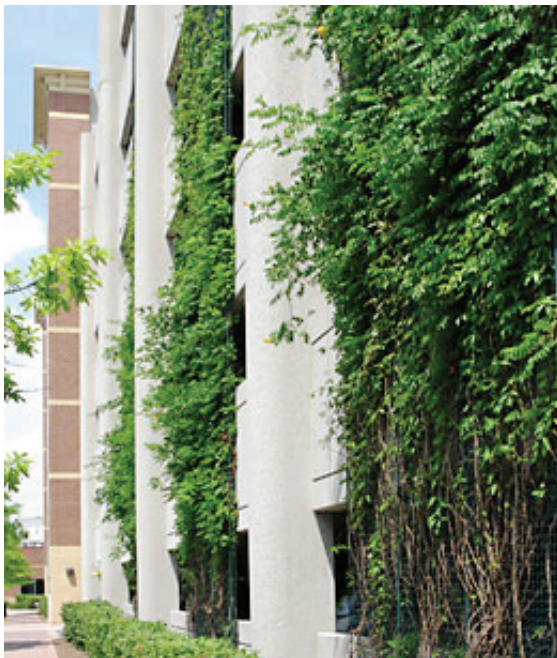
Above left: Several multi-story green walls thrive with correct plant spacing and adequate irrigation and nutrients. Source: greenscreen®
