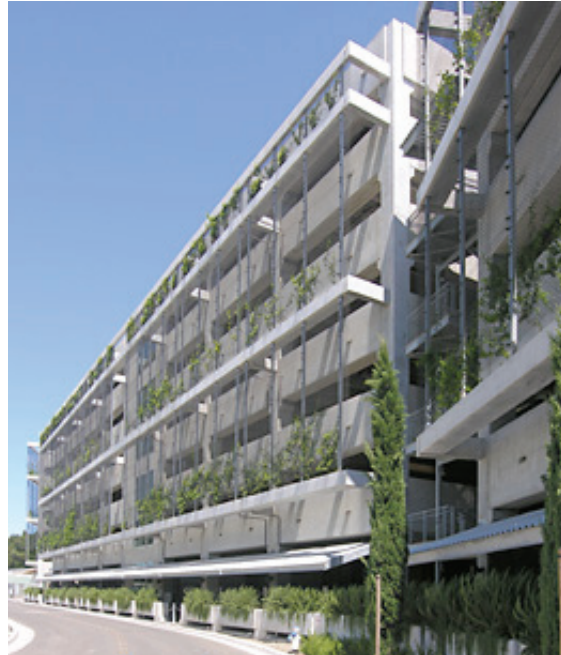
Above: A large multi-level parking structure with a green facade. Source: greenscreen®
